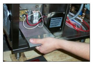
Removing the lower strainer.
